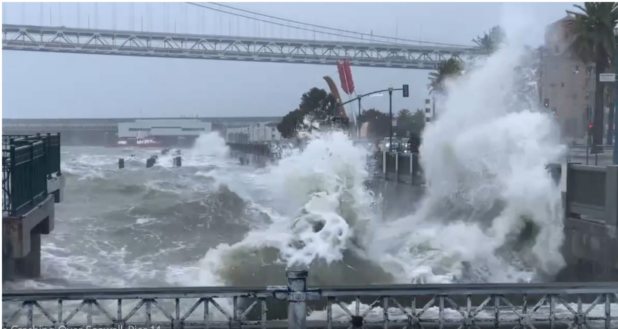
Figure 2-6: Overtopping of Seawall in March 2023
